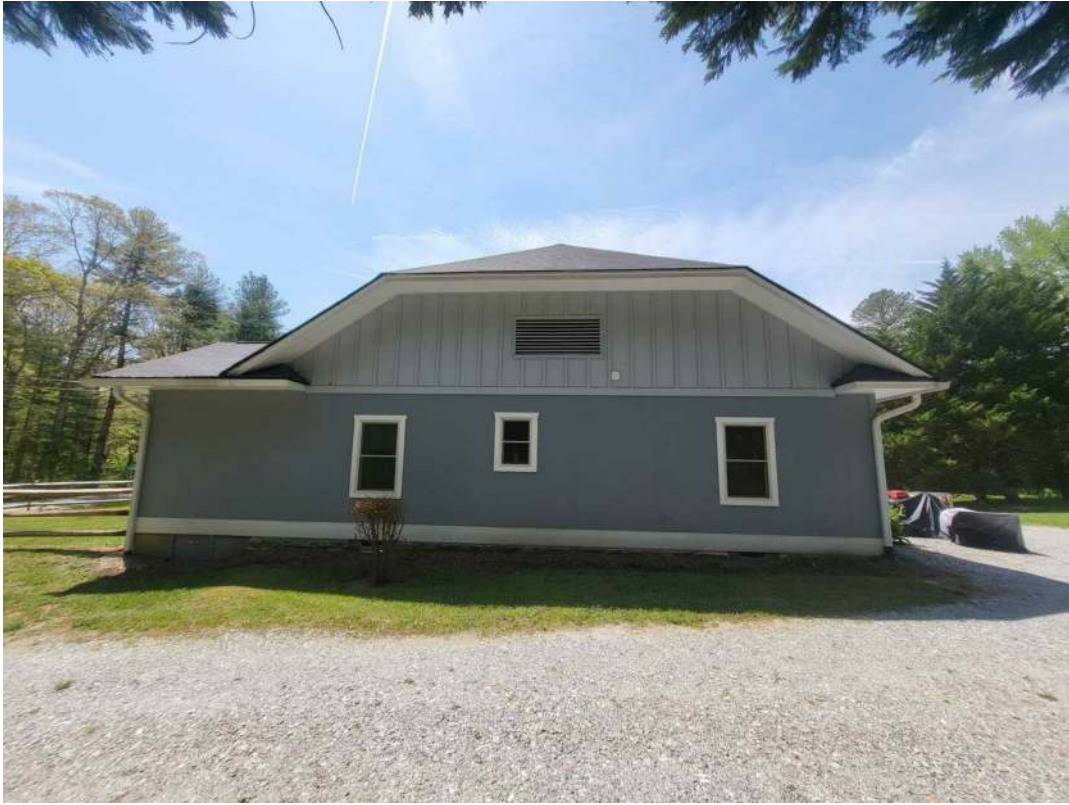
Right Semi Detached - Structure Right Photo
