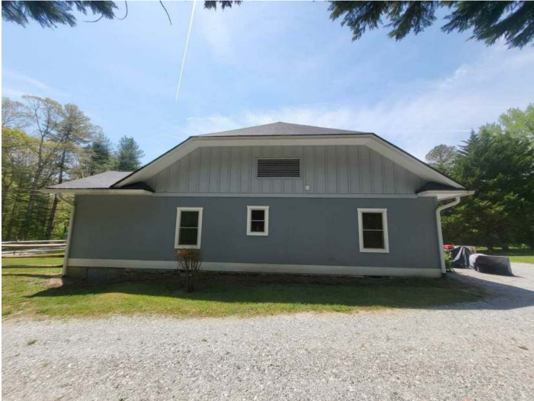
Right Semi Detached - Structure Right Photo
